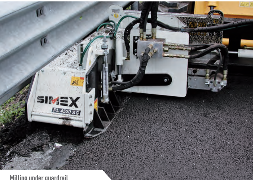
Milling under guardrail
